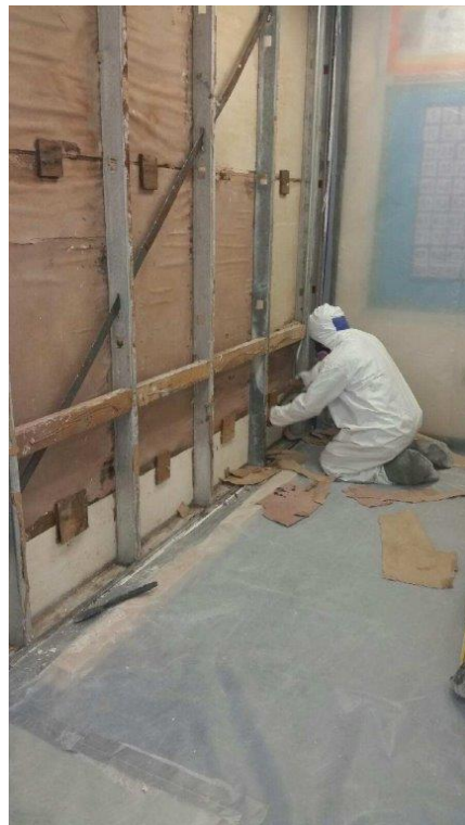
Photo 8: St. John's Lane Room 79 – After Remediation
