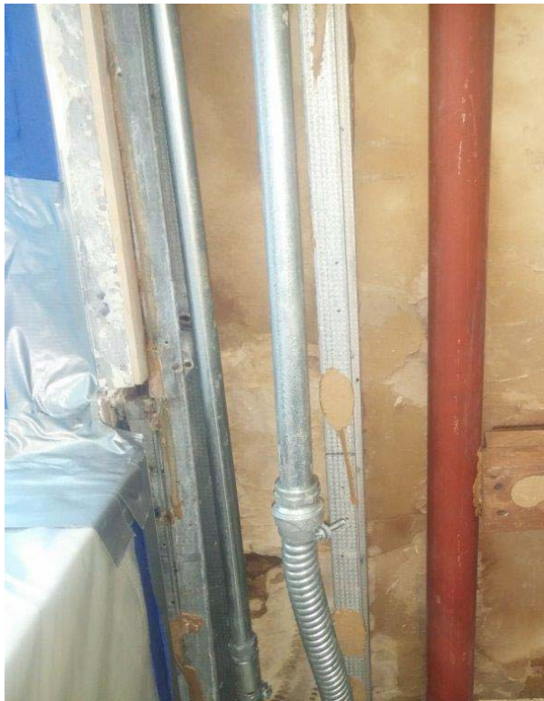
Photo 7: St. John's Lane Room 79 – After Remediation
