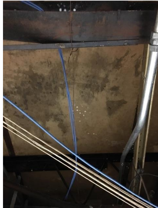
Photo 10: St. John's Lane Library Room 102 Above Doorway – After Remediation
