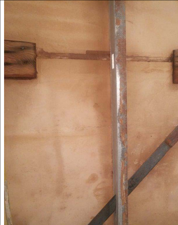
Photo 5: St. John's Lane Room 79 – After Remediation
